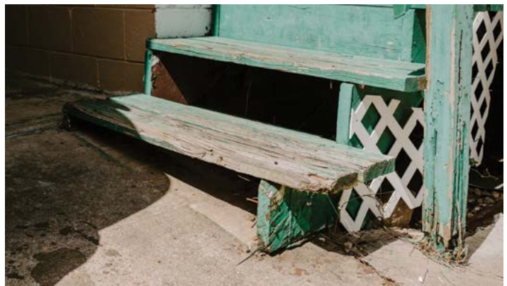
There are nails protruding from the rotting wooden steps leading to the home's front door of Kelley's home.
